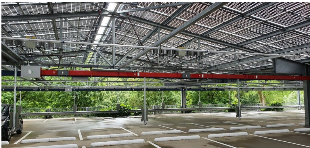
Car Park covered with solar panels; busways connecting to string optimizers
