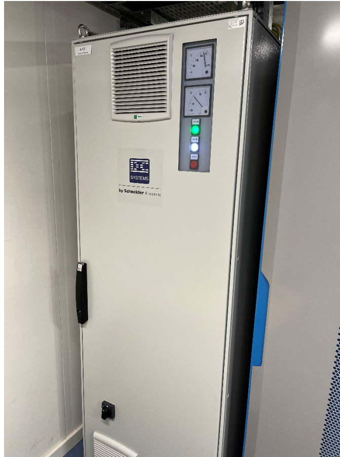
DC Systems Active Front End built by Elektro Internationaal
